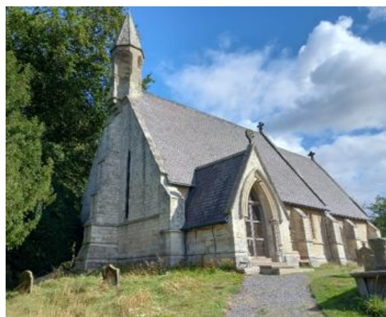
St Wilfrid's Church, South Stainley Source: Geoff Brown
